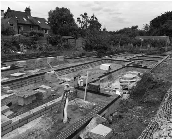
Foundations of the new guest houses
